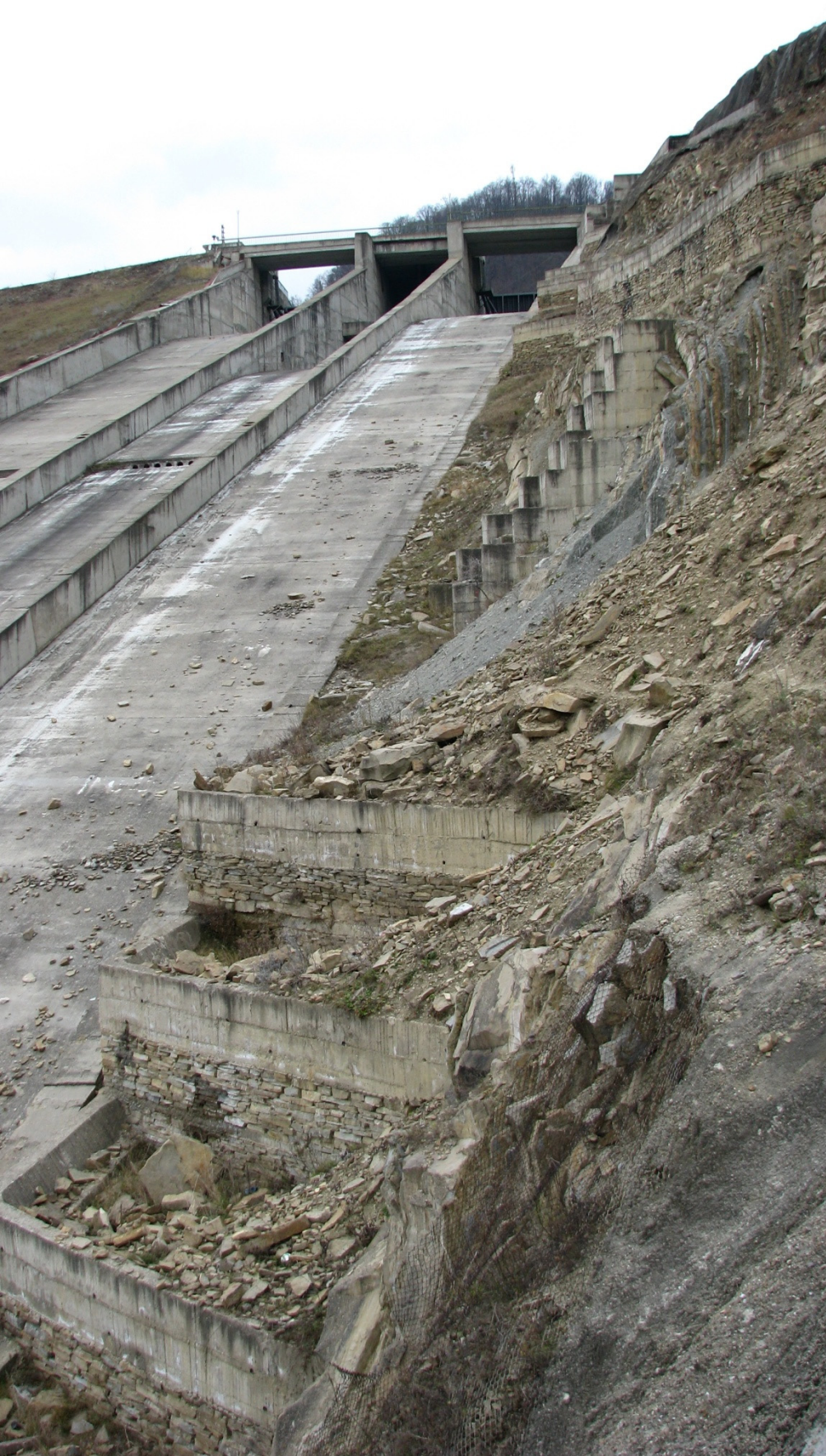
Deformation of the waterdam infrastructure due to the slopes instability
